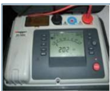
Insulation control with Megger measuring device
