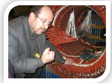
Specific electrical machine inspection
